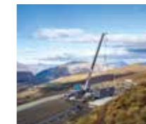
Snow Factory under Construction
